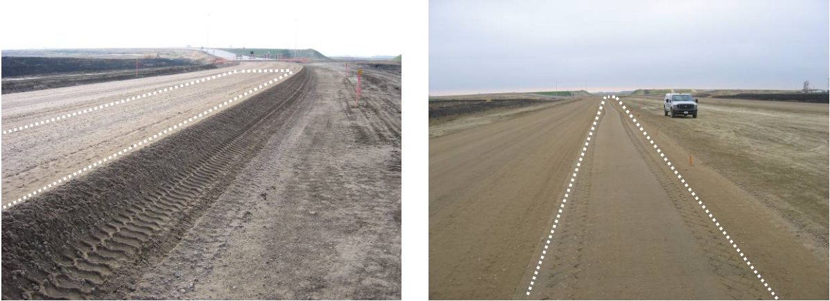
Figure 2.6. Test strip (outlined with dashed lines) comprised of granular material with testing locations spaced at 7.6-m intervals
