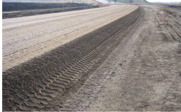
Figure 6.1. Strip 1, comprised of Class 5 subbase material overlying compacted subgrade
