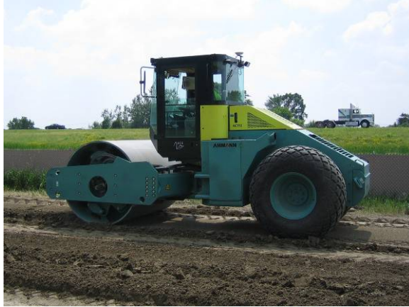
Figure 6.3. Ammann AC-110 vibratory smooth drum roller
