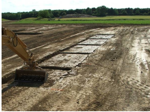
Figure 6.2. Excavation of natural subgrade for construction of Strip 2 with variable lift thickness
